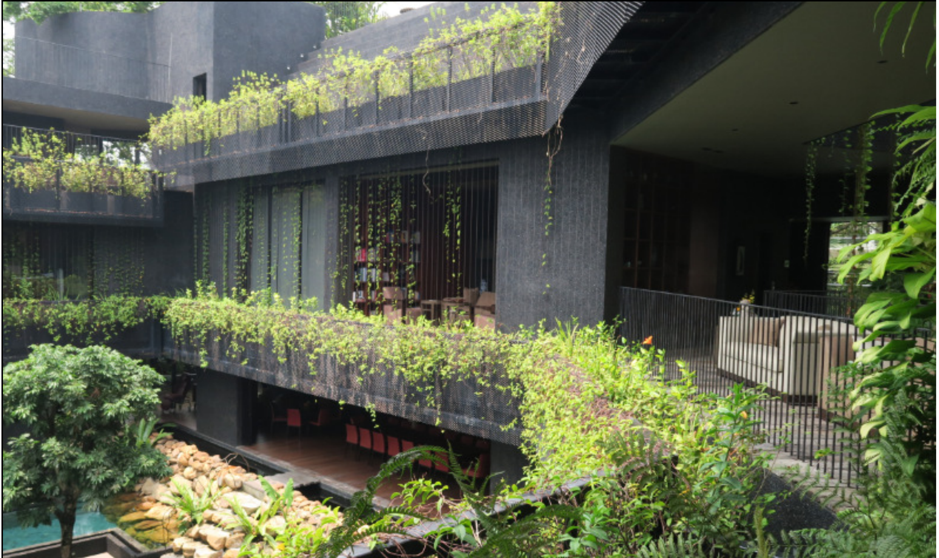
CORNWALL GARDENS ROOFTOP GREENERY
