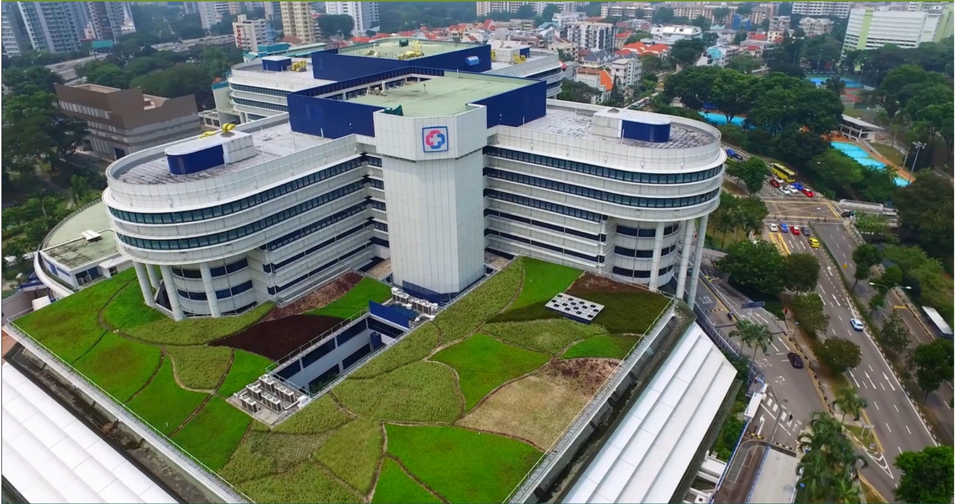
KK WOMEN'S AND CHILDREN'S HOSPITAL ROOFTOP GREENERY
