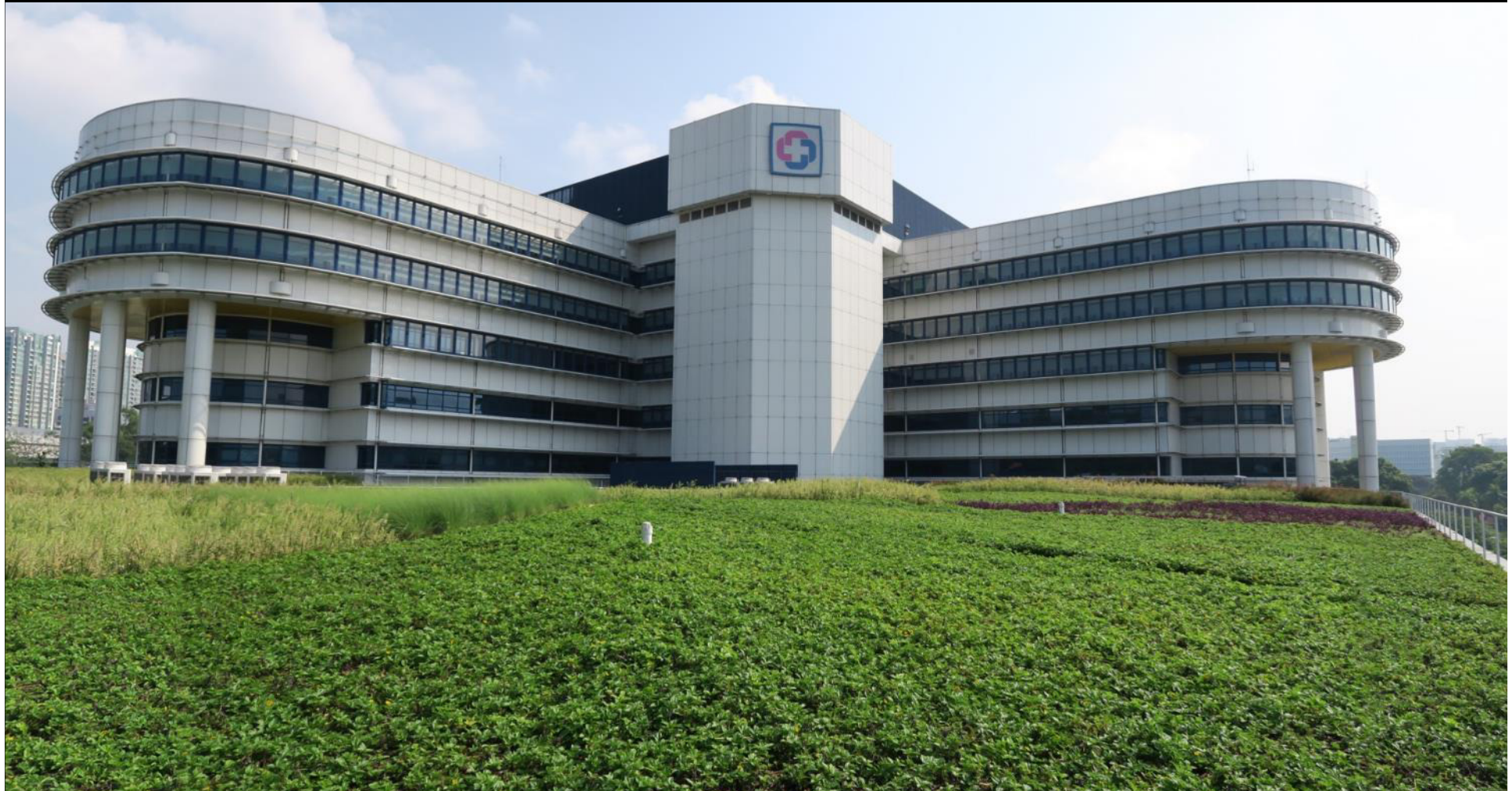
KK WOMEN'S AND CHILDREN'S HOSPITAL ROOFTOP GREENERY
